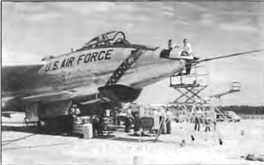
RB-47E, serving as the Monticello I prototype in a photo taken at the Lockheed plant in Marietta. Rome Air Development Center at Griffiss AFB, NY was also a major player in the program. Rome ADC was heavily involved in developing ECM and electronic reconnaissance equipment. This photo was taken of the photo on display at the Marietta museum in very challenging lighting conditions and required Gus Letto's Photoshop expertise to clean it up.
